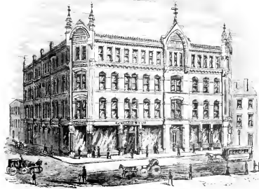
Appleton Bank Block, erected 1875.
