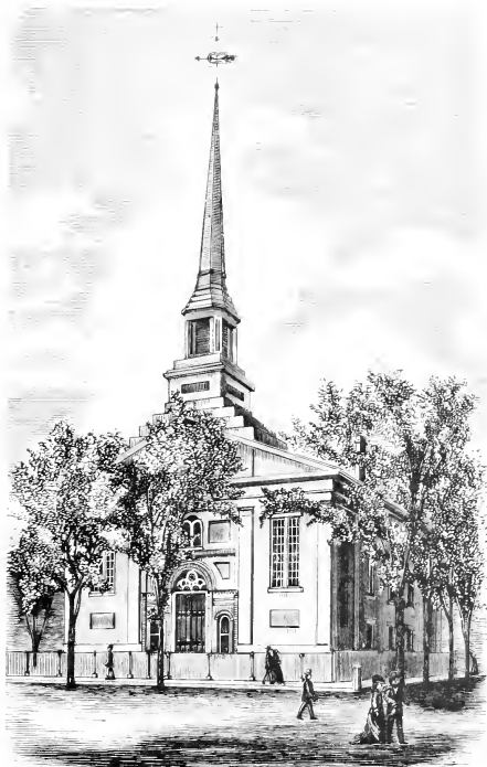
John Street Congregational Church.
