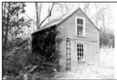
Original setting of Hearse House, Sudbury, MA
